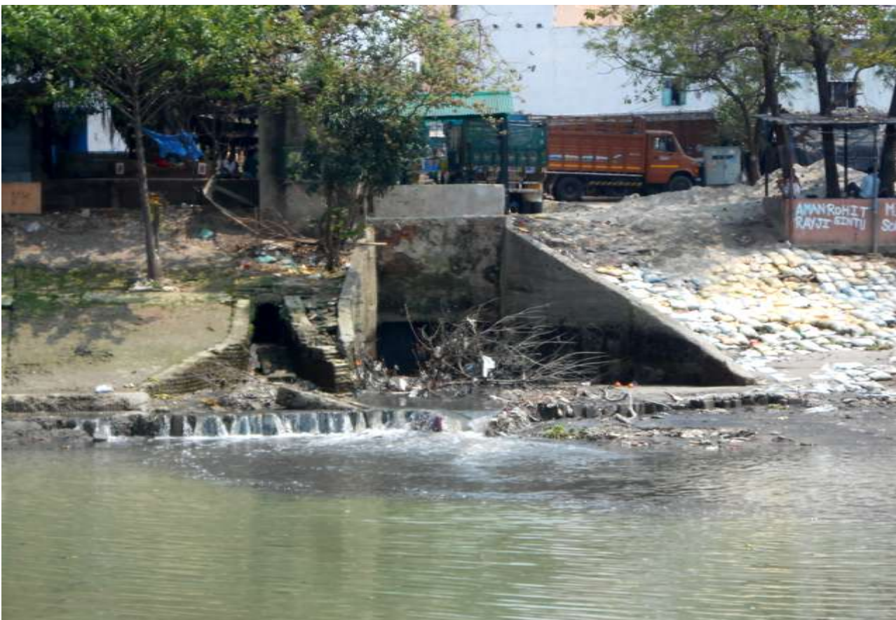
Plate 136– Opening up of Sewer line in Ariadaha area
