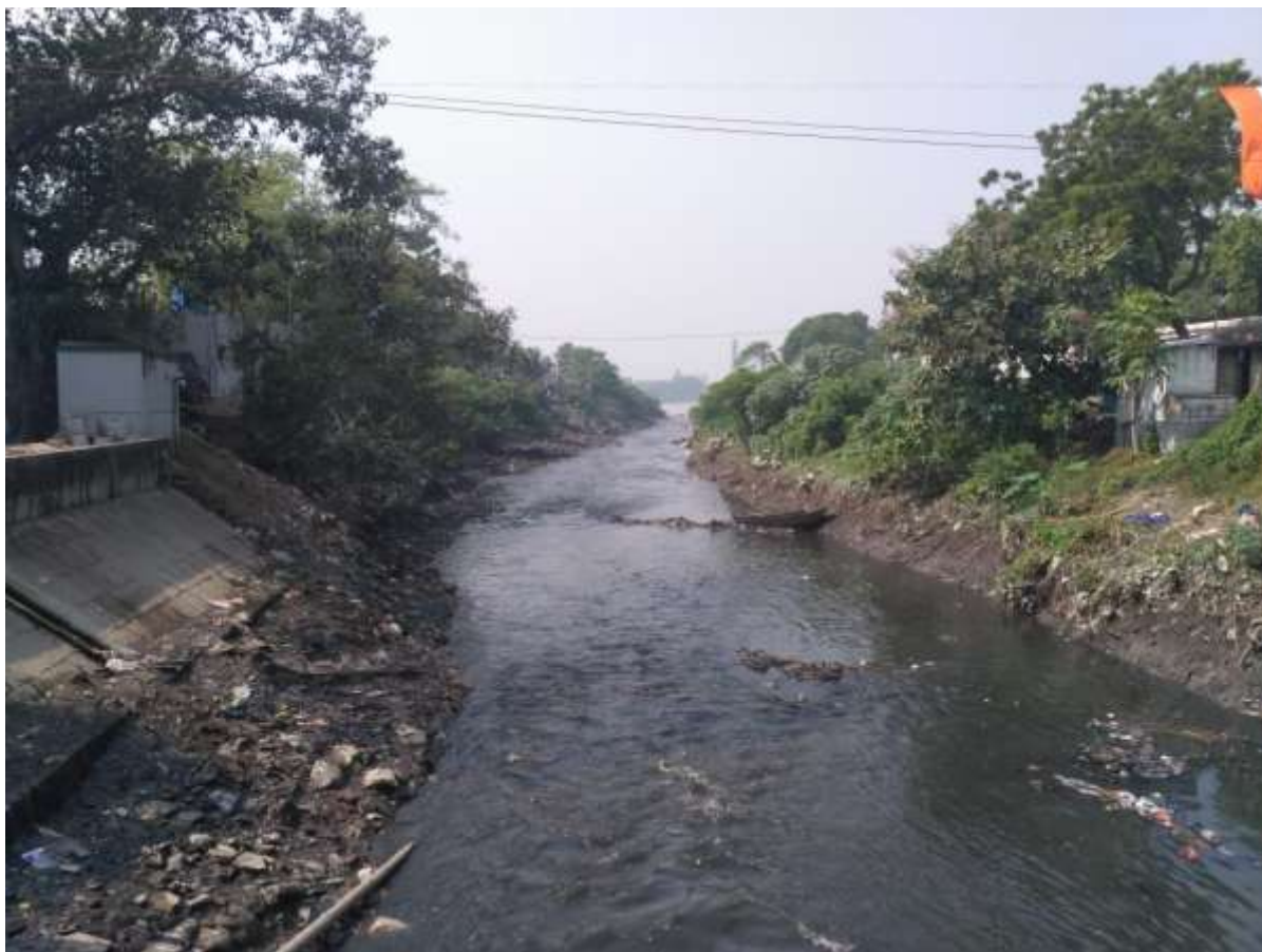
Plate 31– Khardah Khal , 22°43'36.37"N 88°21'42.50"E
