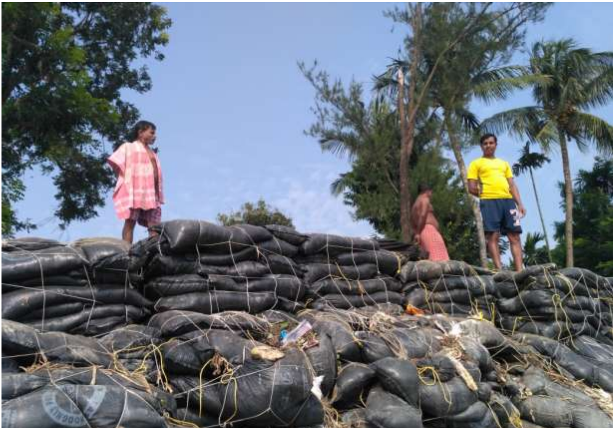
Plate 131 & 132 - Rectangular White Polypropylene Non Woven Geo Bags filled with sand are used for Bank Protection , Near Nimtala Ghat , Garulia Municipality .
