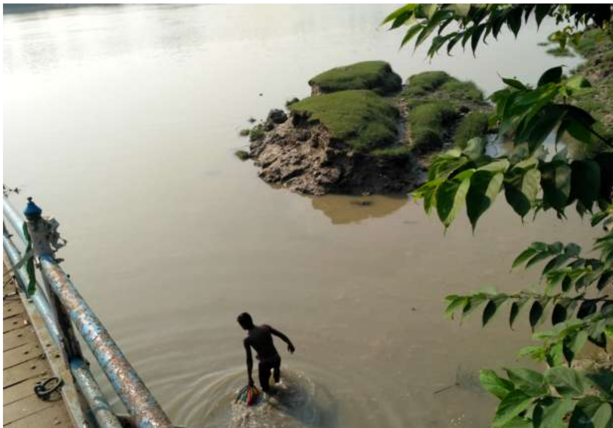
Plate 121- RKG Brick Kiln, near Anthpur Ferry has been inundated
