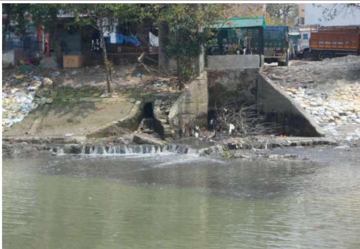
Plate 32 –Drain Line near Ariadaha , Kamarhati Municipality
