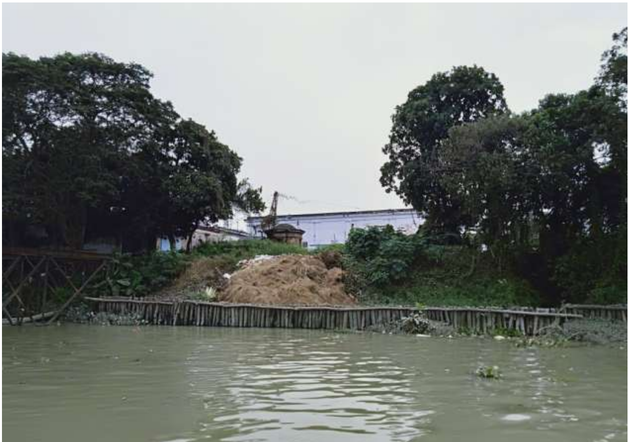
Plate 126– Logs are used to check bank erosion , Bhatpara Municipality, 22°51'32.80"N 88°22'30.77"E ,
