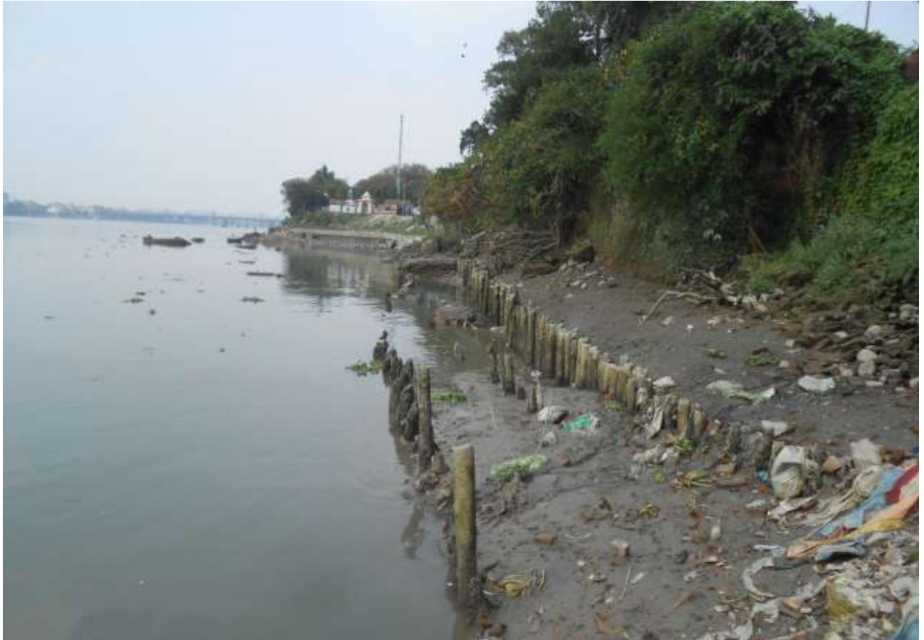
Plate 127– Logs are used for checking Bank Erosion , Kamarhati Municipality , 22°38'59.93"N 88°21'30.79"E
