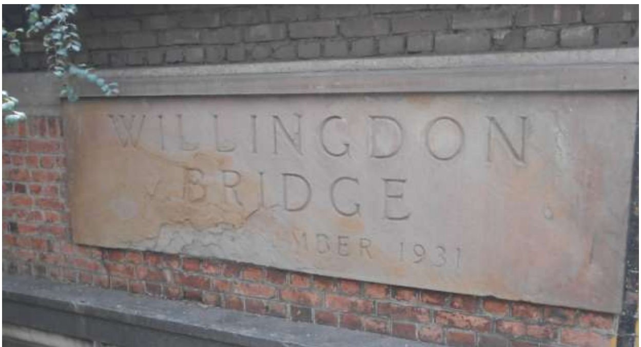
Plate 72- Willingdon Bridge , Plaque in Vivekananda Bridge
