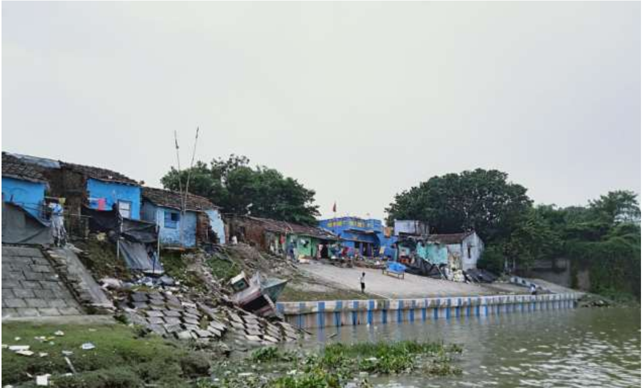
Plate 125– Breach of Embankment in the Shyamnagar area , Garulia Municipality, 22°49'42.68"N 88°22'36.28"E
