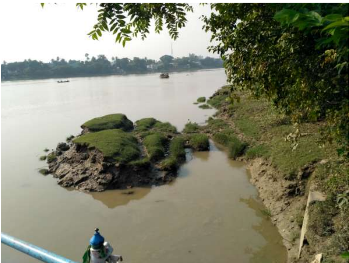
Plate 134– Collapsed river Bank near Anthpur Ferry Ghat , 22°50'37.69"N 88°22'34.54"E
