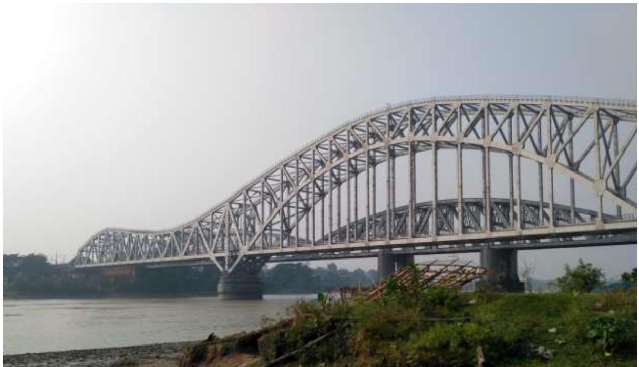
Plate 75 – Sampreeti Bridge on River Hugli.
